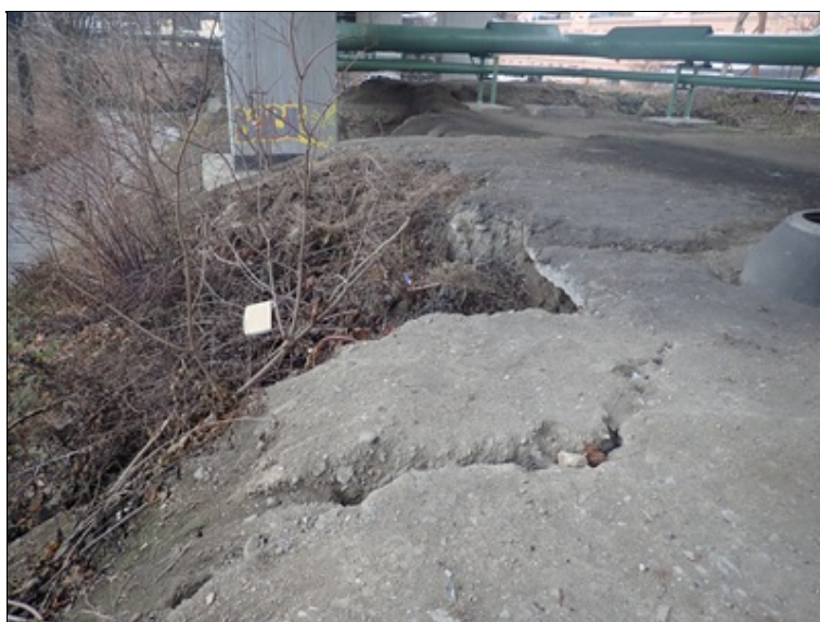
Detail eroze svahu
