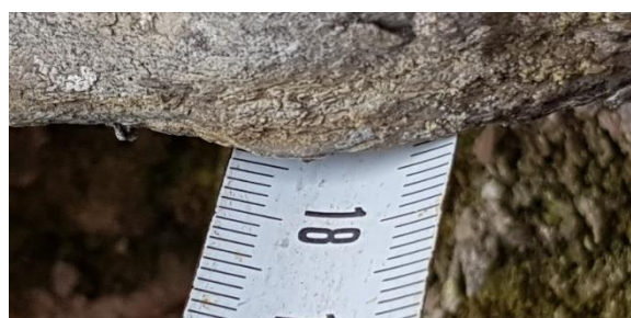
Obr. 13 – Dtto obr. 12 – Hloubka kaverny cca 175 mm
