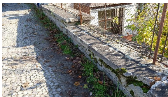
Obr. 05 – Dtto obr. 04, uchycená vegetace ve sparách.
